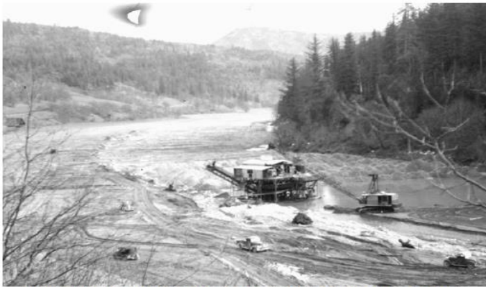
Looking down Horse Creek, just above confluence with Middle Creek. Circa 1940
