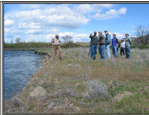
Photo 5. Eroding sandy streambank in need of riparian-wetland vegetation's stabilizing influence.
