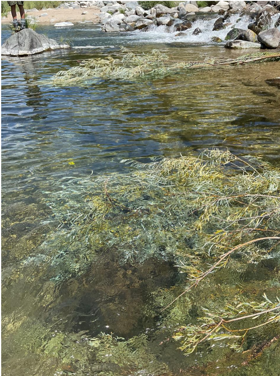
Photo 8. Brush bundles added to the Kelsey/Scott mixing zone. August 3, 2023.
