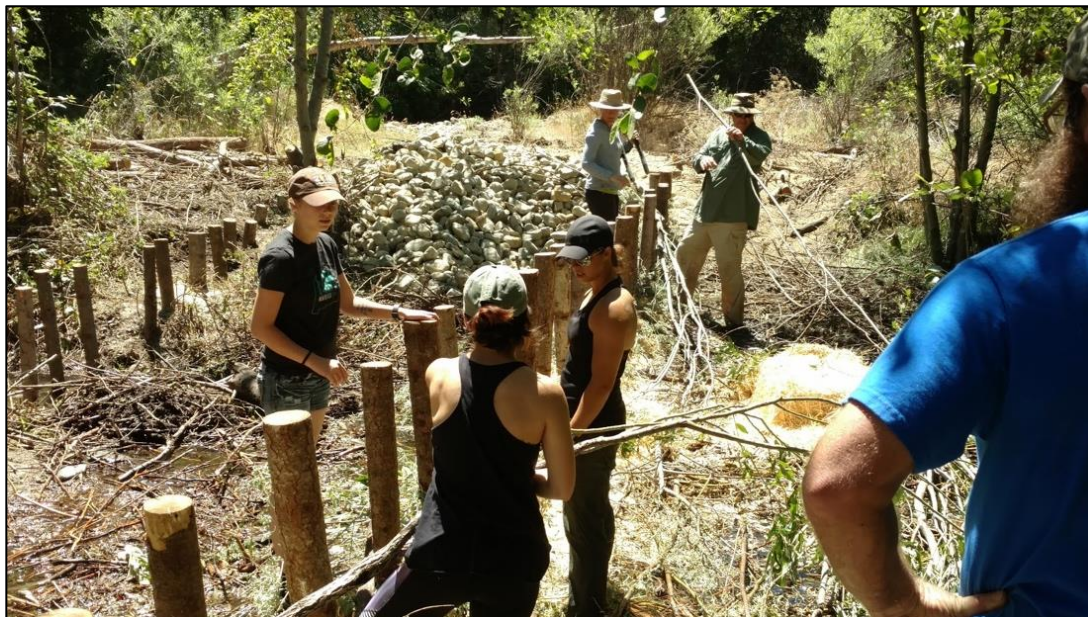
Figure 31. French Creek Beaver Dam Analogue 1 during construction. Photo taken 6-21-2017.
