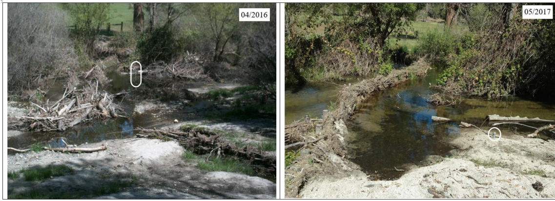
Figure 32. Miners Creek Feature Photos. Left photo: significant breach of BDA and draining of pond. Note location of ground water well with pipe extending approximately 5 feet above channel bed. Right photo: Significant aggradation behind repaired BDA one year later. Note location of same ground water well with pipe extending approximately one foot above channel bed.
