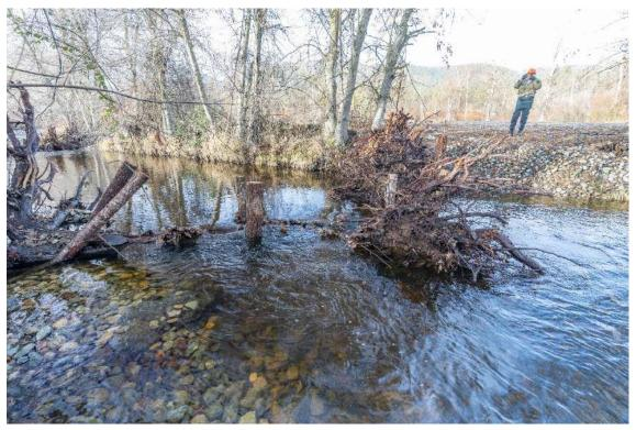
Photograph 8. Channel Spanning Wood Structure
