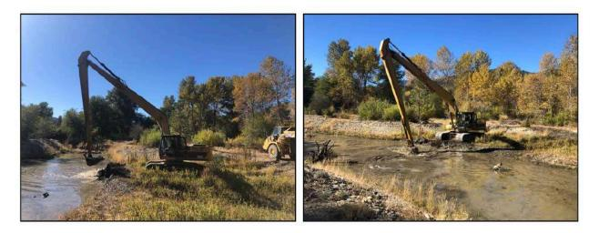
PHOTO 7. REMOVAL OF SEDIMENT IN THE SIDE CHANNEL, OCTOBER 15, 2020.
