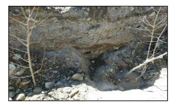
Photo 3. Cottonwood poles planted at a depth of  $\sim$ 10' into groundwater - March 2018.
