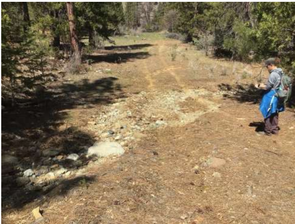
Photo 2.11: Gully 2 crosses road again. EFR13.1. April 13, 2023.
