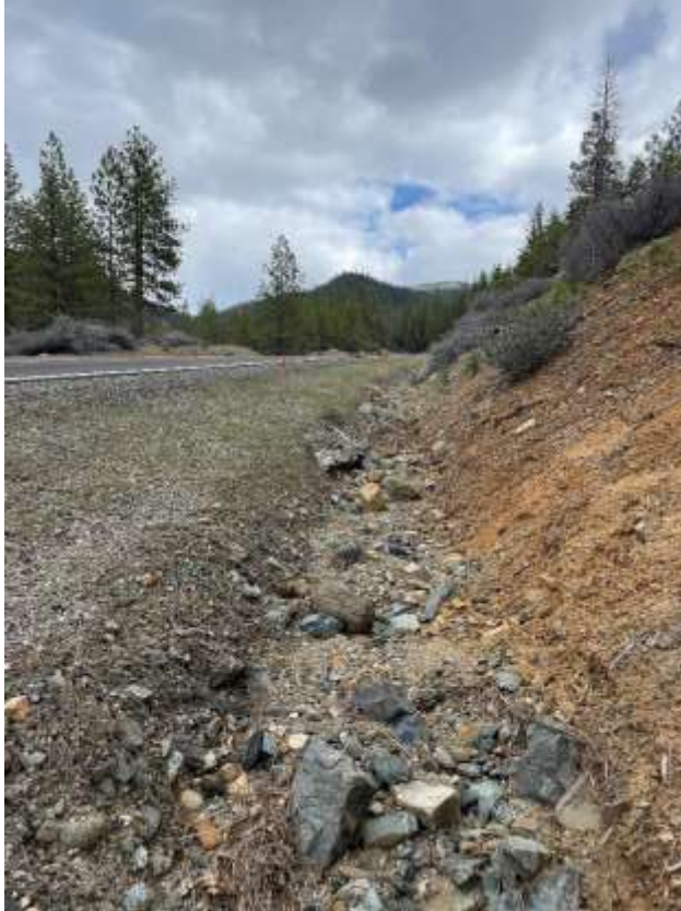
Photo 2.50: This inboard ditch on Highway 3 is the source for EFG 24. EFG24a. April 5, 2024.
