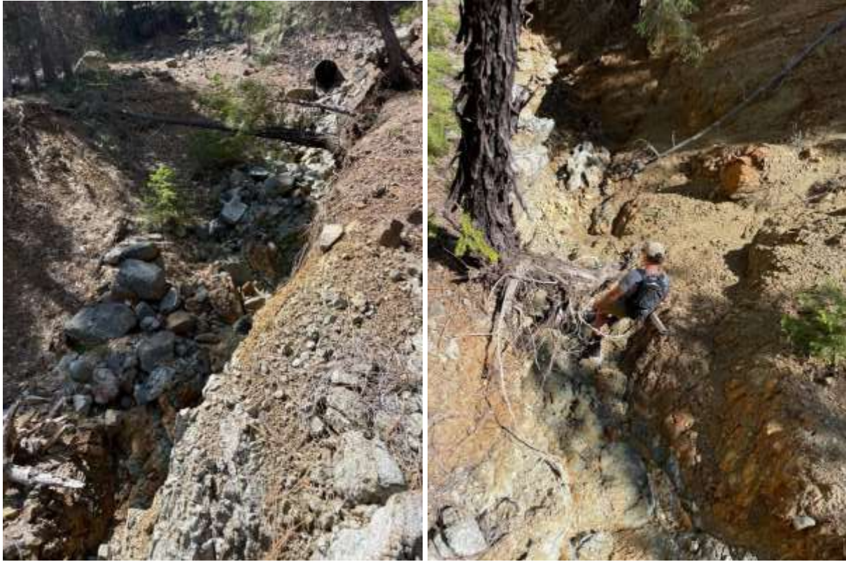
Photos 2.22 and 2.23: Left, culvert discharging in Gully 8. EFG8f. Right, Beginning of deep incision. EFG8f. May 29, 2023.
