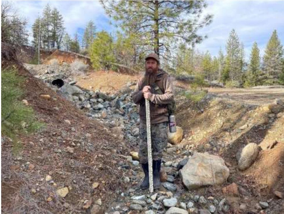
Photo 2.4: Outlet of Highway 3 culvert, looking upslope. EFG2a. January 19, 2024.
