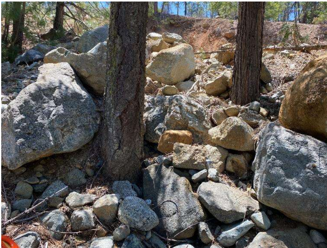
Photo 2.15: Below Highway 3 outboard ditch. EFG6.5.2c; June 2, 2023.
