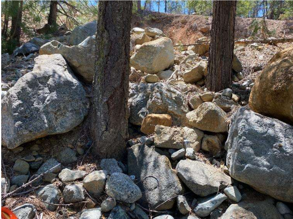
Photo 2.45: Below Highway 3 outboard ditch. EFG6.5.2c. June 2, 2023.
