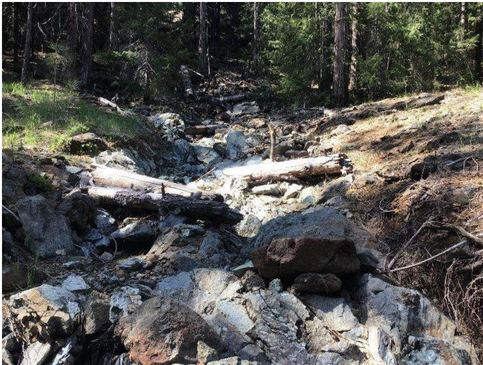
Photo 2.36: Discharge from outboard ditch erodes fill at the top of Gully Complex 12. January 18, 2024.
