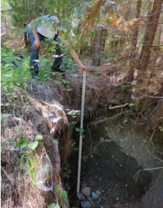
Photo 2.1: Gully Complex 49, upslope reach. EFG49g. July 25, 2023.
