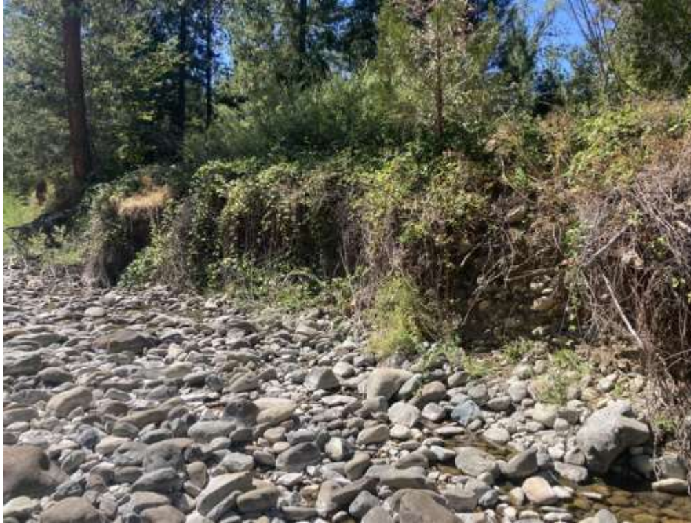
Upstream end of RKM 5.0 cutbank
