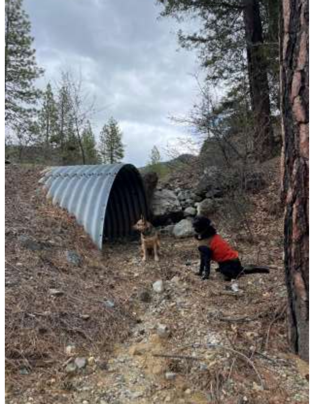
Photo 2.51: Beginning of EFG 24. Inboard ditch flows past culvert. EFG24a. April 5, 2024.
