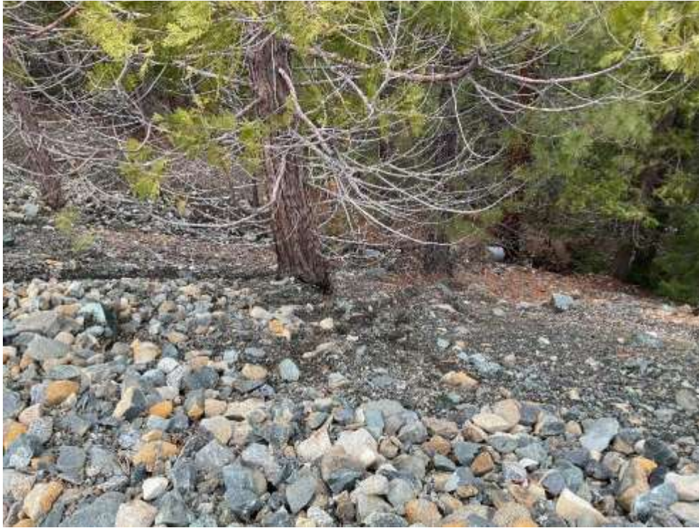
Photo 2.35: Culvert discharges at the top of Gully Complex 12. January 18, 2024.
