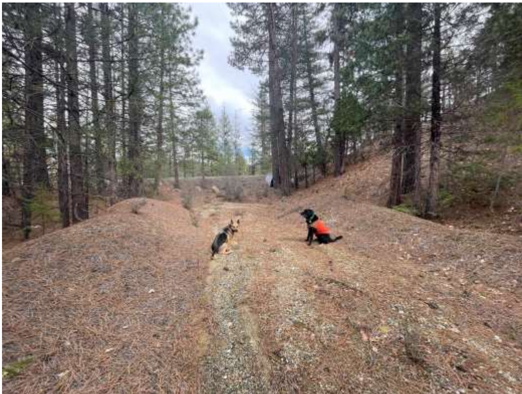
Photo 2.18: EFG 24 downstream of bypassed culvert. April 5, 2024.
