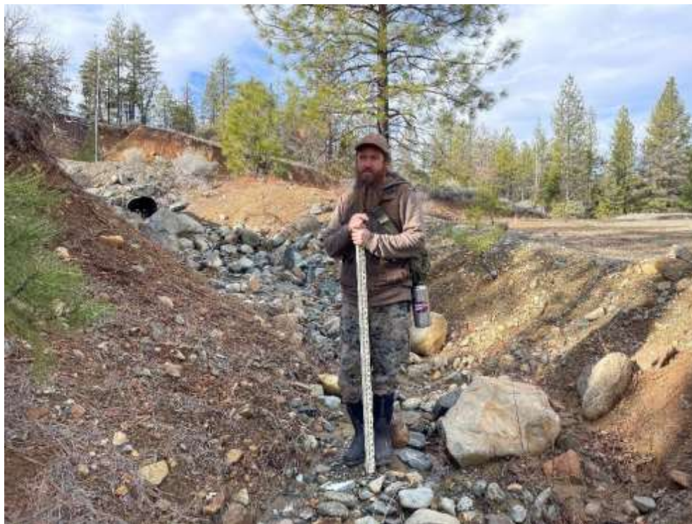
Photo 2.6: Outlet of Highway 3 culvert and ditch, looking upslope. EFG2a. January 19, 2024.
