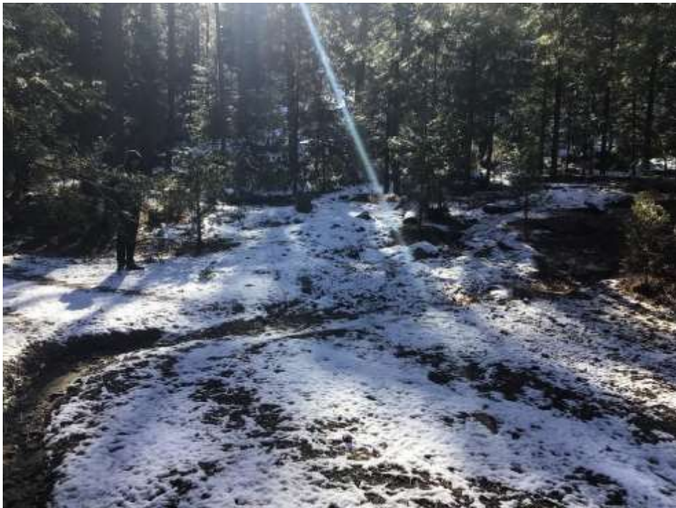
Photos 2.17 & 2.18: Gully Complex 2 crossing lower road. EFR13. January 20, 2023.
