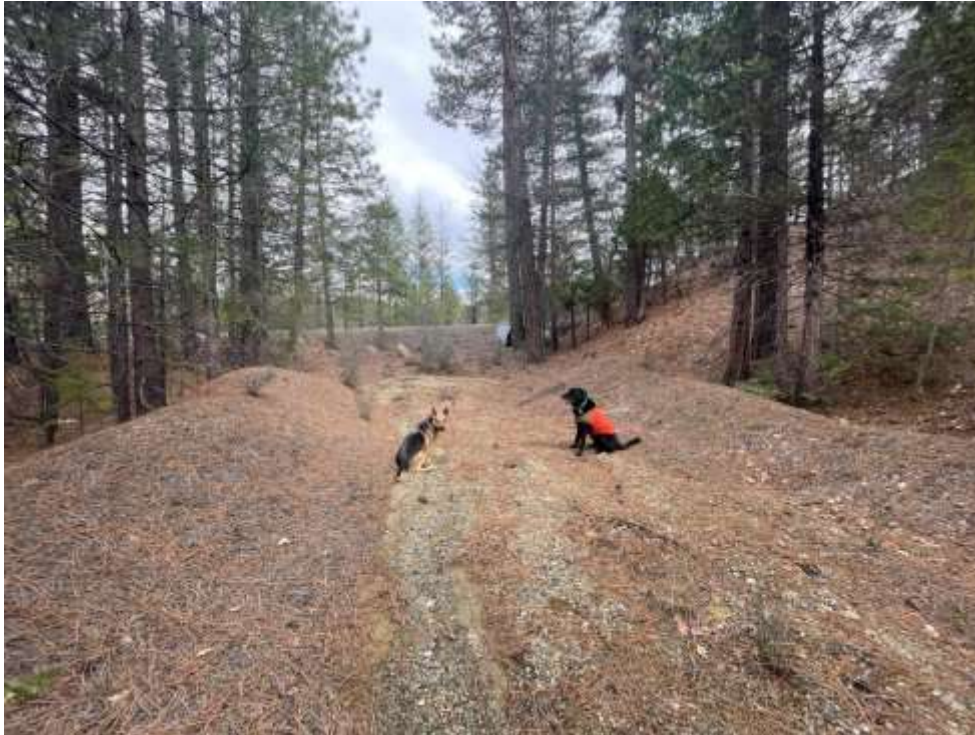
Photo 2.52: EFG 24 downstream of bypassed culvert. April 5, 2024.
