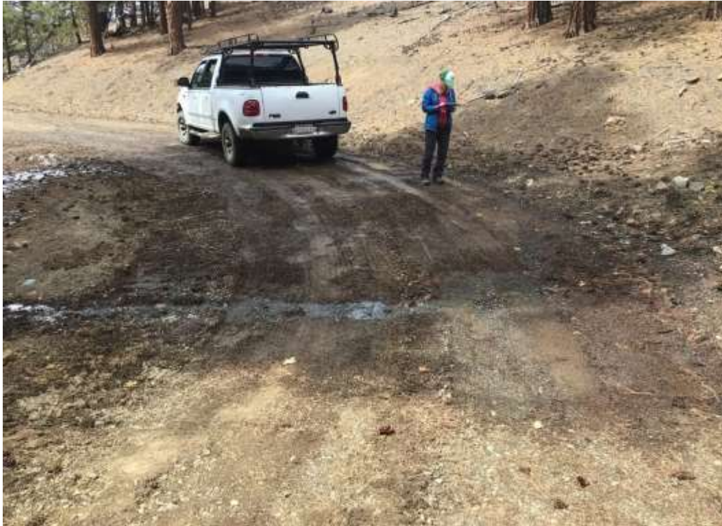
Photo 2.1: Example of mild erosion point. HRR20, April 18, 2023.
