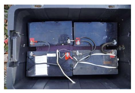
Picture 9. Example of battery bank setup at array site.
